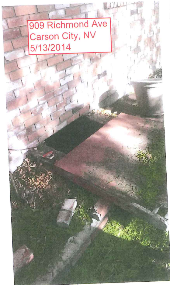
BACKVIEW CRAWL SPACE
