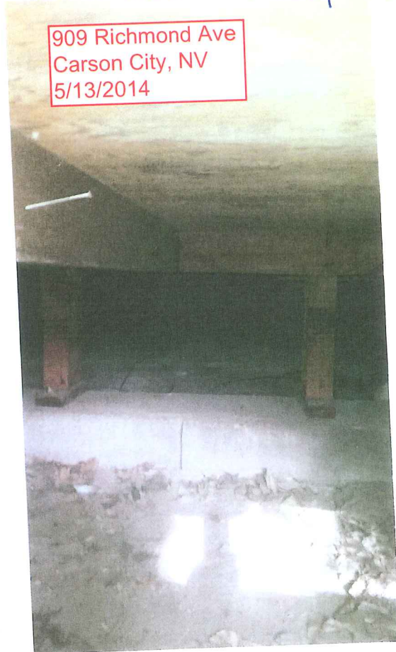
BACK VIEW - CRAWLSPACE
